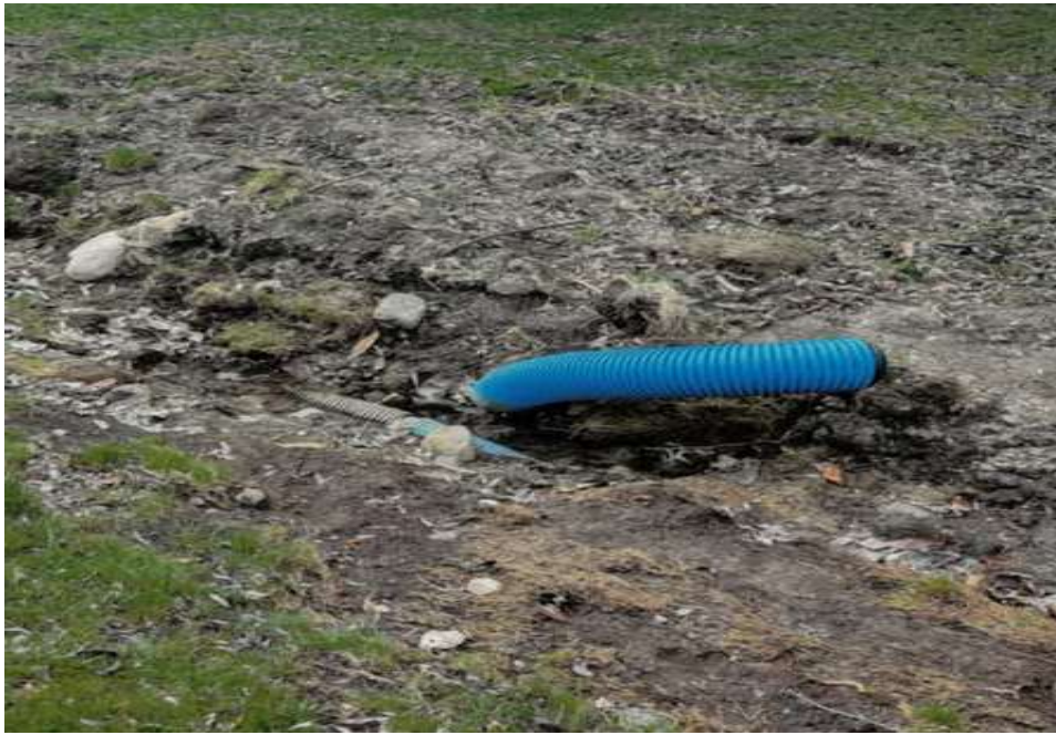
South Catch Basin
